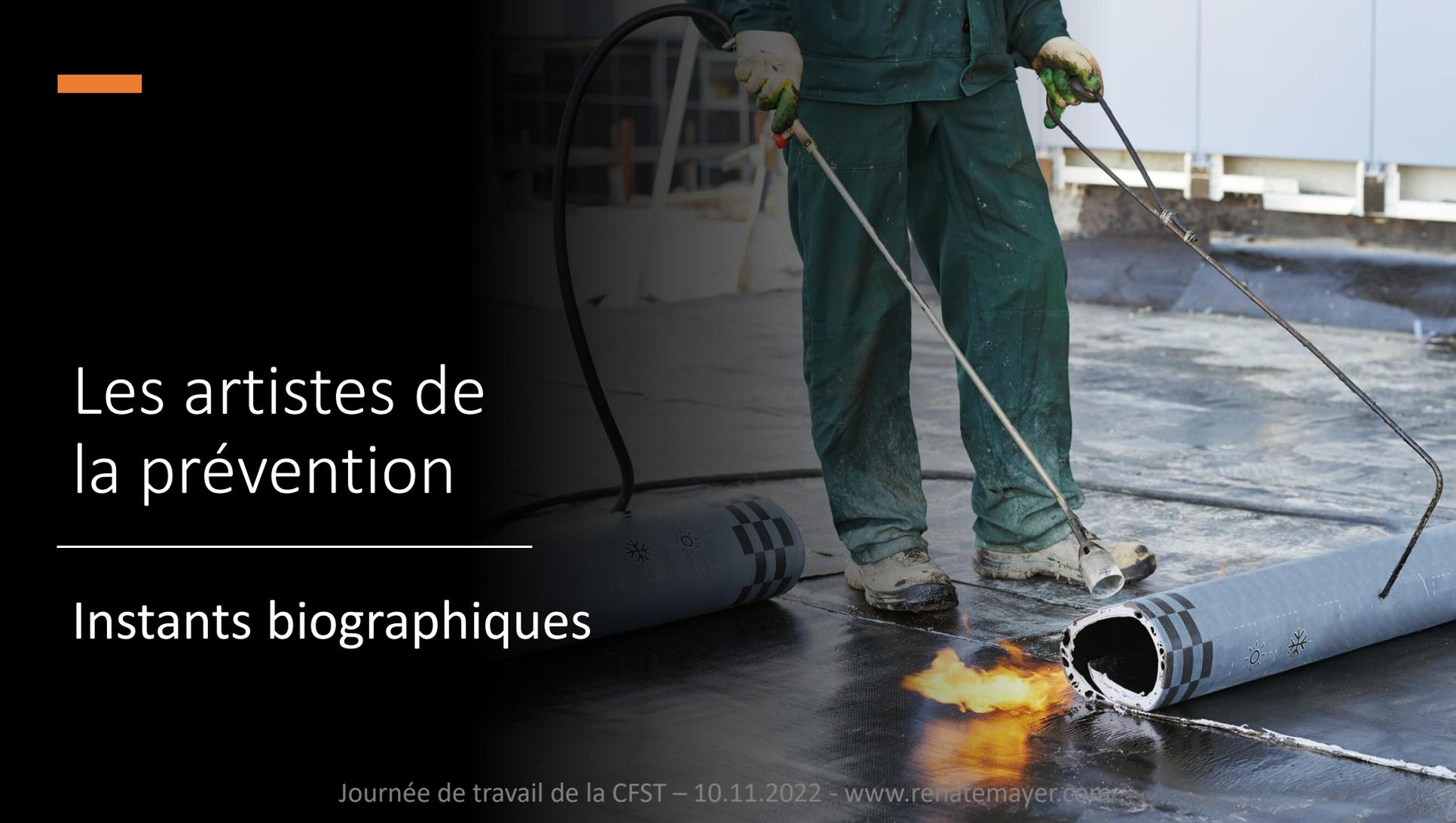
A worker wearing green protective overalls and gloves is using a torch to heat a roll of material on a construction site. The worker is standing on a dark, reflective surface, possibly a roof or a large sheet of material. The torch is held in the worker's right hand, and the roll of material is being heated by the flame. The background shows a construction site with various structures and materials.
